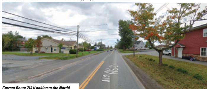
Current Route 214 (Looking to the North)
