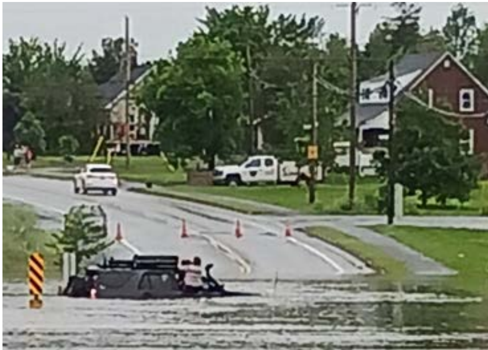
Figure 2: Highway 2 Crossing Over Barneys Brook – 2023-07-22 (Client Provided)
