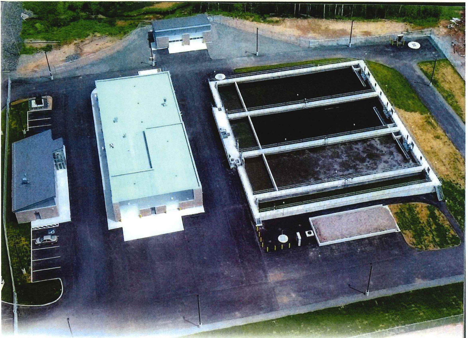
Cape Breton Regional Municipality (CBRM) adopted a user fee and cost recovery model to provide wastewater services in a sustainable and affordable manner. Photo: Sydney Harbour West WW Treatment Plant courtesy of CBRM
