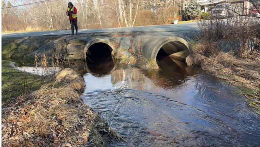
Photo 7: Outlet of two twin 1050 mm concrete culverts under Poplar Dr
