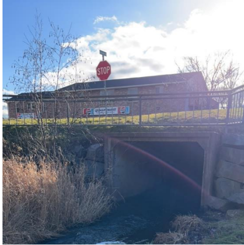
Photo 4: Inlet of 2100 mm X 1800 mm concrete box culvert under Highway 2
