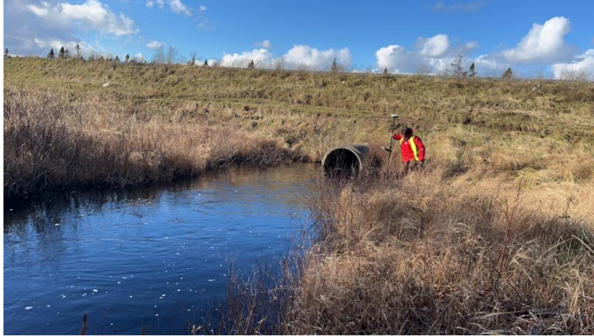
Photo 10: Outlet of 1050 mm concrete culvert under Highway 102
