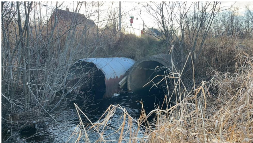
Photo 3: Inlet of twin CSP and concrete 1200 mm diameter culverts under Church St
