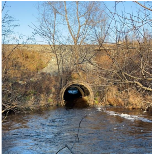
Photo 2: Outlet of 1500 mm diameter concrete culvert under Railway just upstream Paley Road
