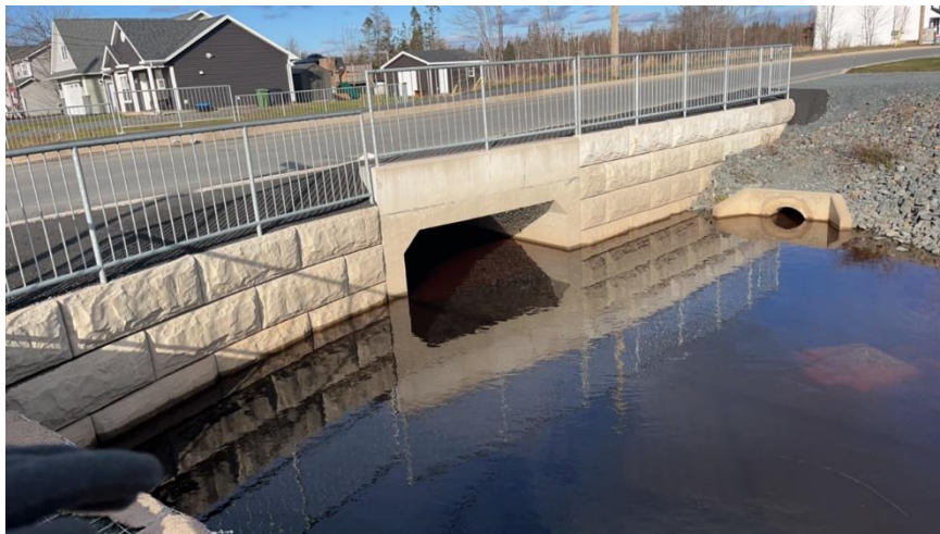
Photo 9: Outlet of 2700 mm X 1350 mm concrete box culverts under Mariah Dr
