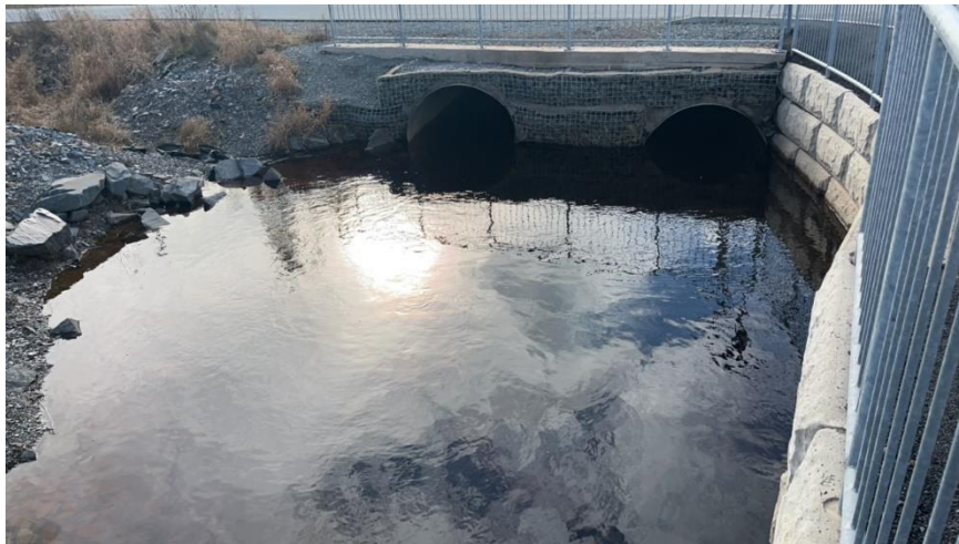
Photo 8: Inlet of two twin 1800mm X 1200 mm CSP ellipse culverts under Turner James Ave
