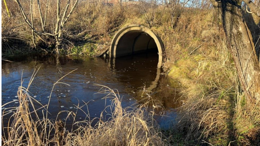
Photo 1: Outlet of 1500 mm diameter concrete culvert under Paley Road
