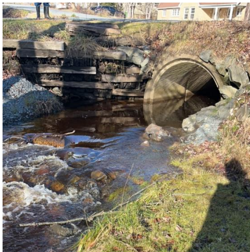
Photo 6: Outlet of 1800 mm concrete culvert under Logan Dr
