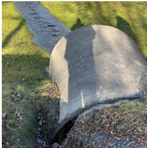
Photo 5: Inlet of 1800 mm diameter concrete culvert under Towerview Ct
