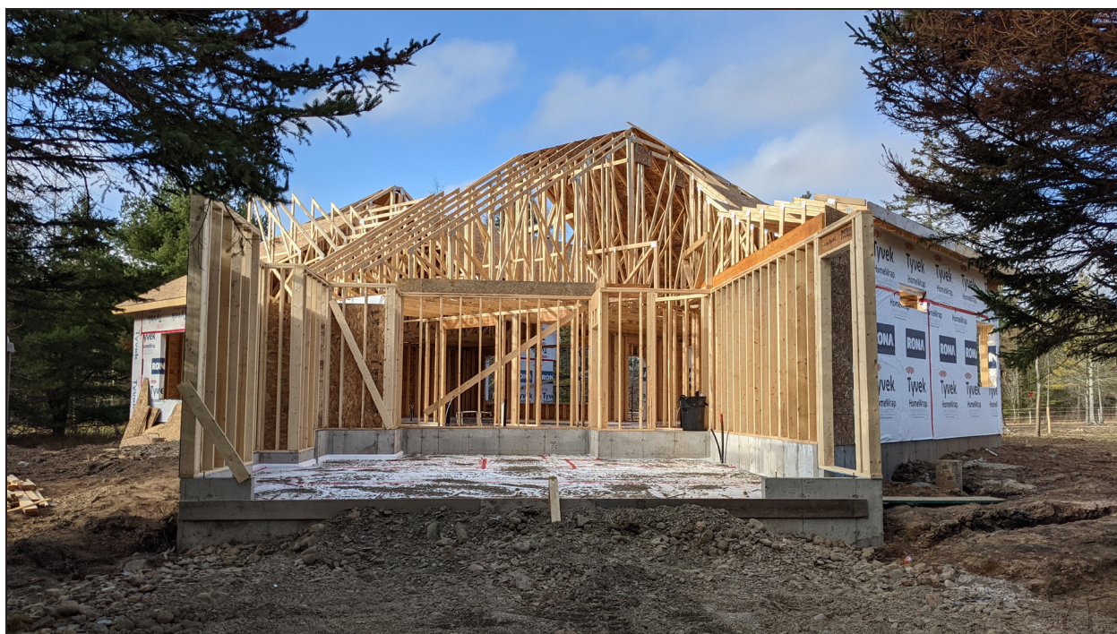
Image 8 - Wood frame of a new house
