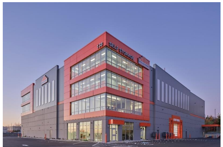
An example of a multiple-storey self-storage building in Bayer’s Lake, NS.
