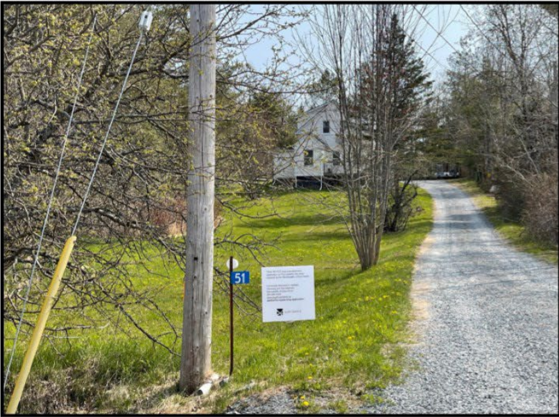
Subject Property—51 Old Enfield Rd.
