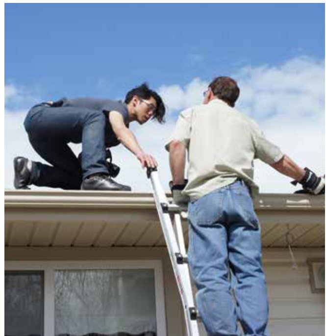
Figure 15: Neighbours remove debris from eaves troughs to reduce risk of home ignition. Courtesy FireSmart Alberta, 2023.
