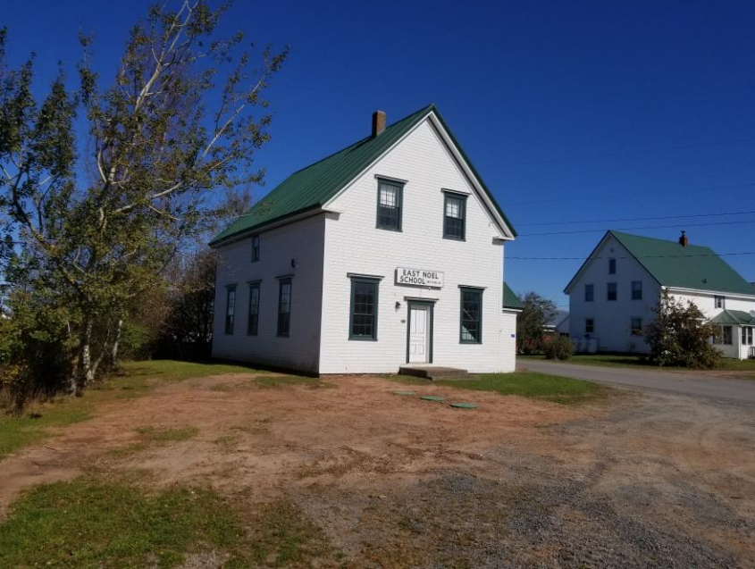
New roof - East Noel Heritage School House
