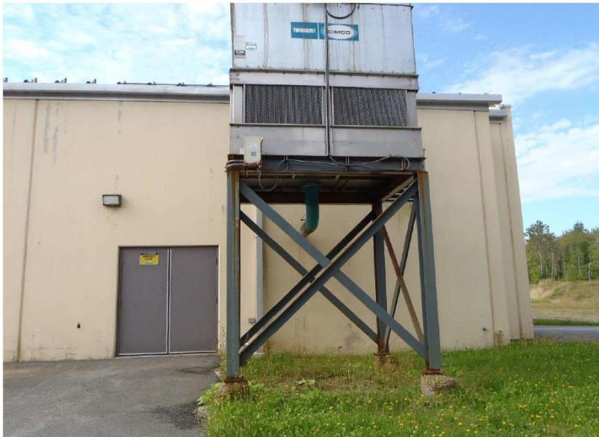
Photo A7 - Steel tower structure
