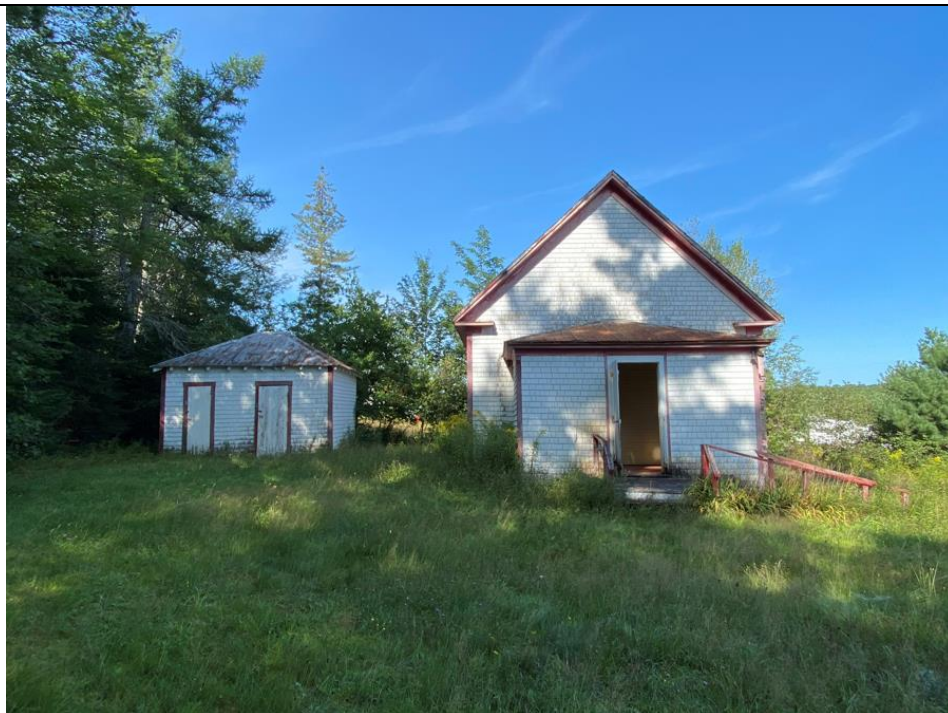
Exterior view of former school building and accessory building
