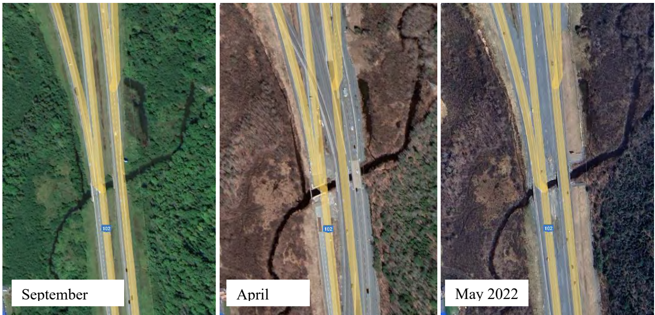
Figure 13 Temporary realignment of Hwy 102 at Site 2.
