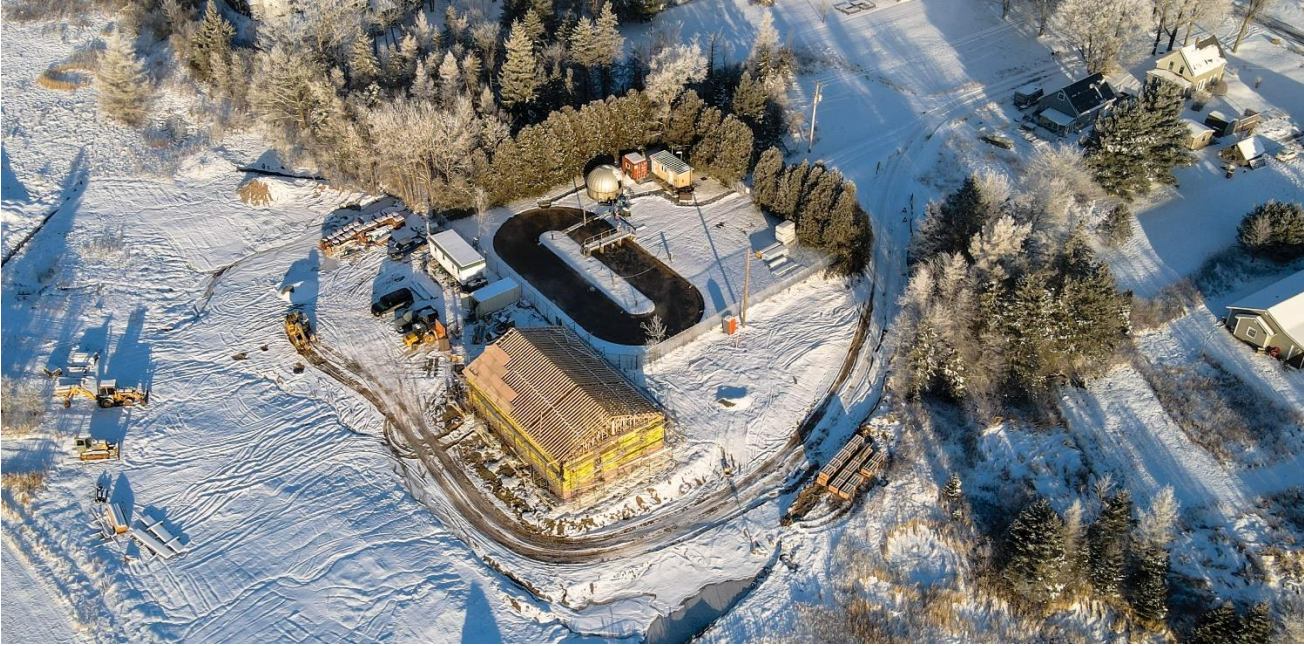
Shubenacadie Wastewater Treatment Plant Construction
