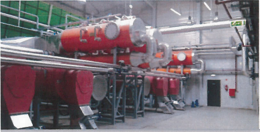
Interior of facility:
