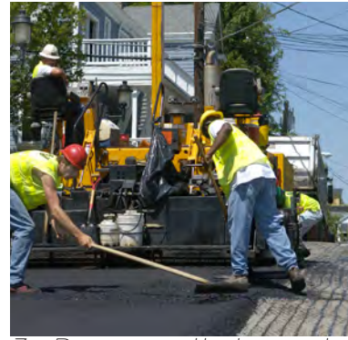
3 - Repave potholes and areas of pooling water
