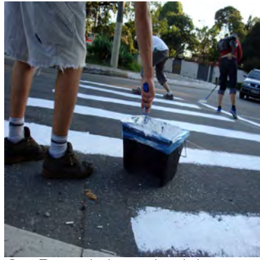
2 - Repaint pedestrian crossing
