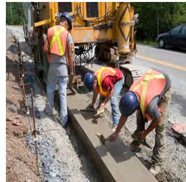
2 - Paving shoulder and/or sidewalk
