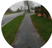
1. Existing Curb and Gutter Sidewalk
