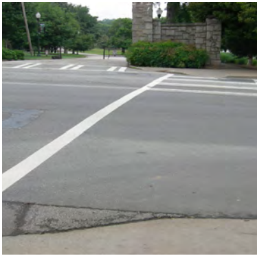
1 & 2 - Improve and repaint markings
