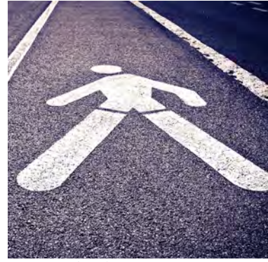
3 - Pedestrian zone pavement marking
