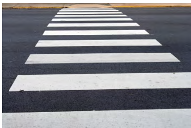
1 - New pedestrian crossing
