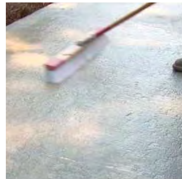
4 - Resurfacing where needed
