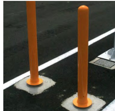
6 - Temporary barriers for pedestrian zone
