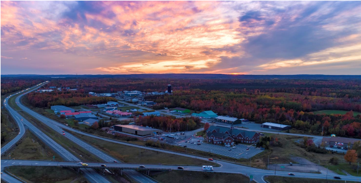
Elmsdale Business Park
