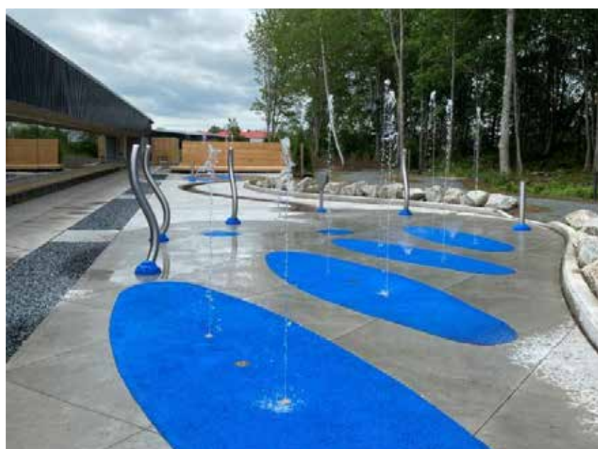
Splash Pad Completed July 2020 - WIP at March 31, 2020
