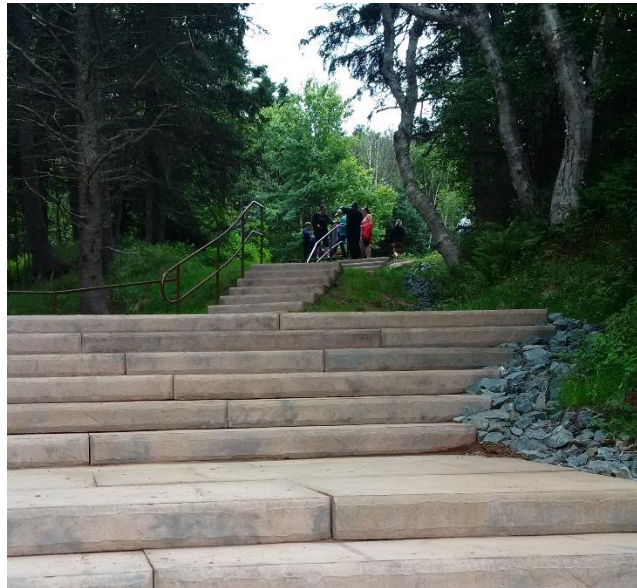
The stairs at Burntcoat Head Park were constructed in 2015/2016 and lead tourists to the ocean floor.
