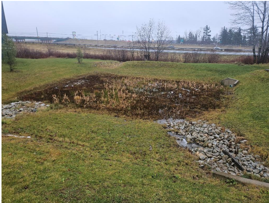
Ph 6 - Above ground storm management area.
