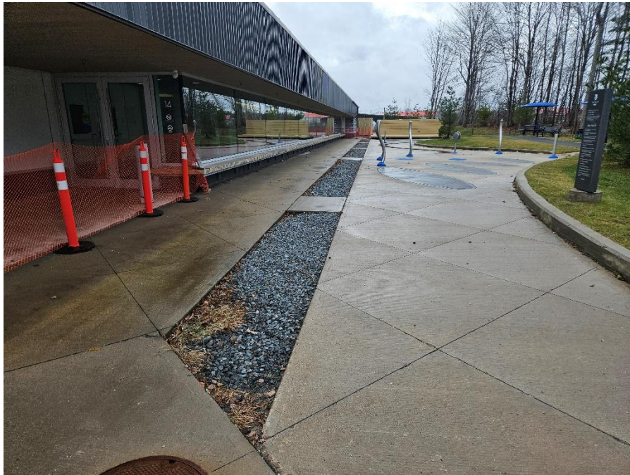
Ph 4 - Existing infiltration trench, to be modified. Trench to be finished with concrete to match surrounding surface.
