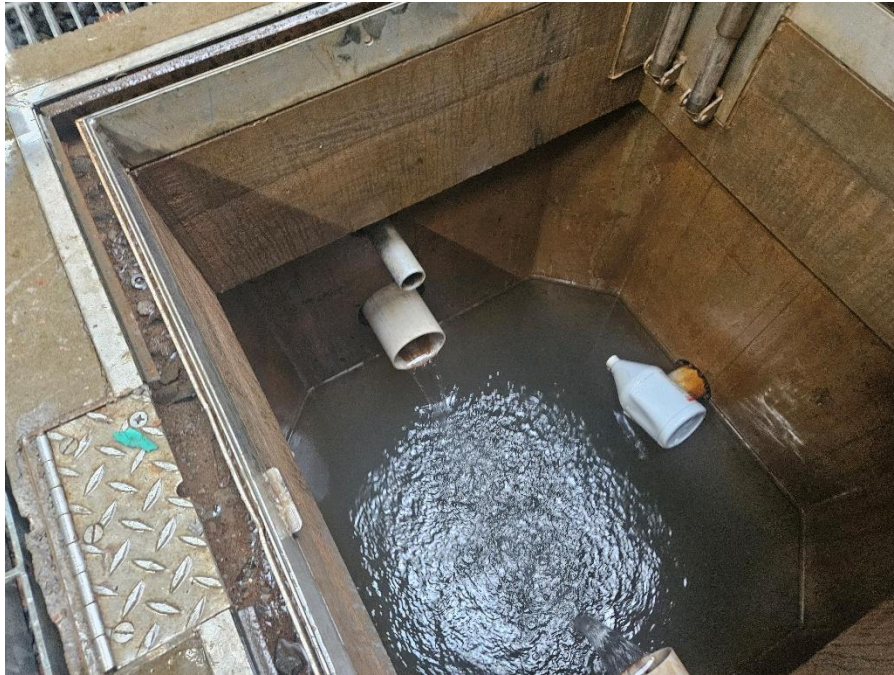
Ph 7 - Sand settling pit.
