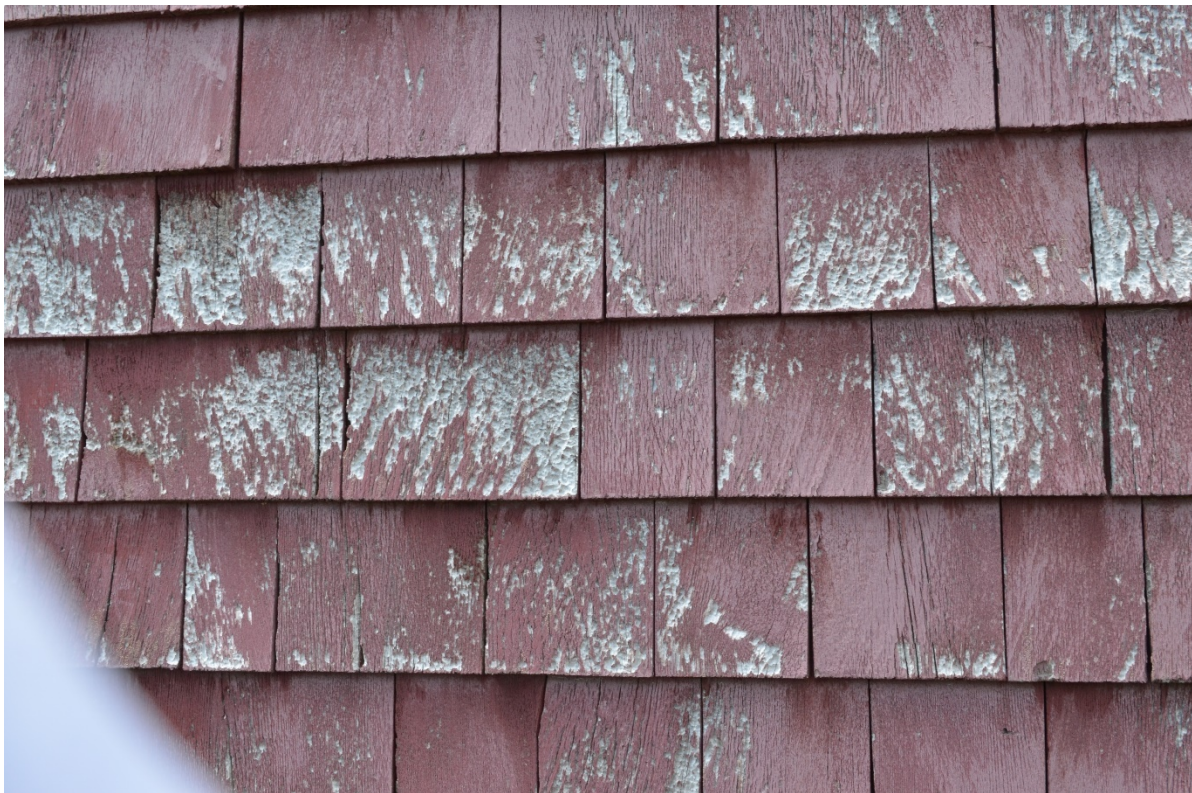
Figure 14: Close-up of shingle damage, driveway side
