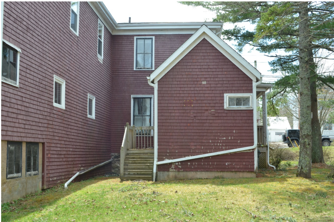
Figure 8: Rear View, Centre Section. Note that eavestrough on narrow section has custom joint and that eavestrough carries sump pump hose. It would have to be removed and reinstalled after painting.
