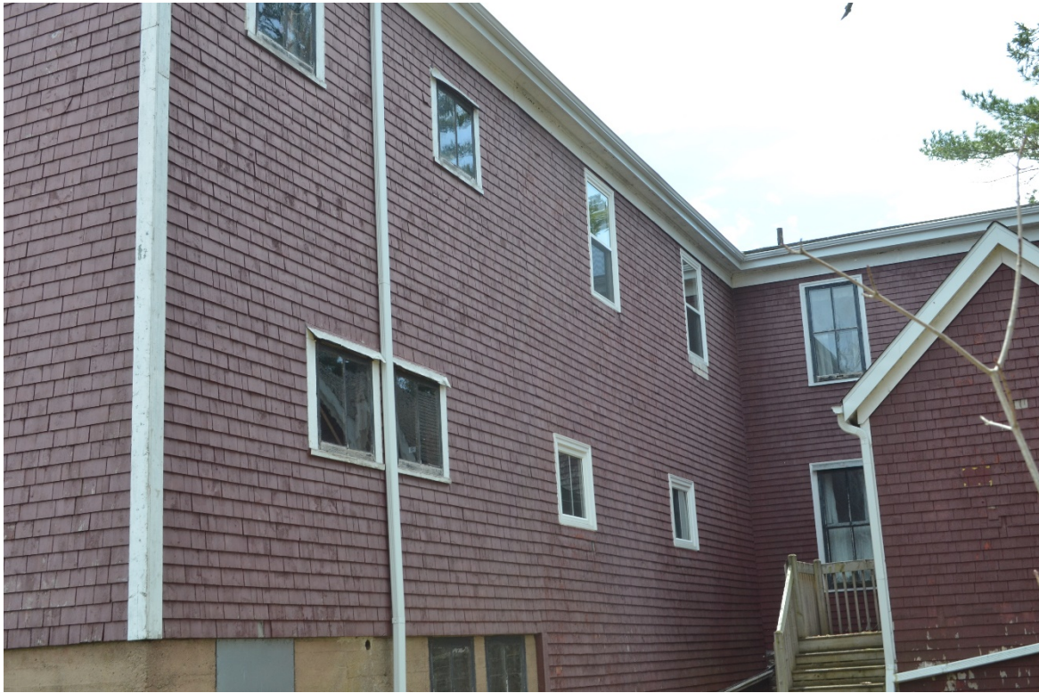
Figure 8: Rear View, Centre Section. Note that eavestrough on narrow section has custom joint and that eavestrough carries sump pump hose. It would have to be removed and reinstalled after painting.
