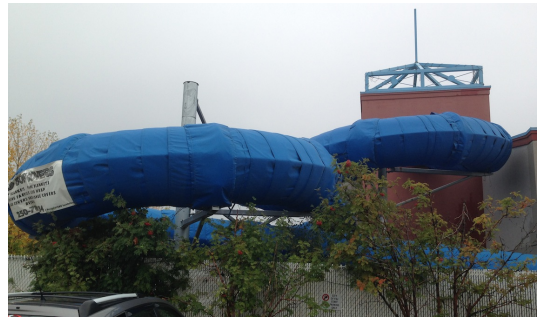
Exterior flume with custom insulated jacket in Fort St. John BC
